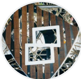
Totally twisted: facade elements overhead
