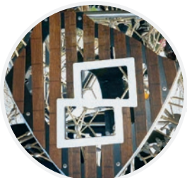
Totally twisted: facade elements overhead
